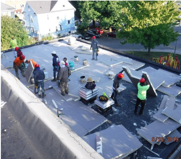
School #33 – Roofing replacement project
