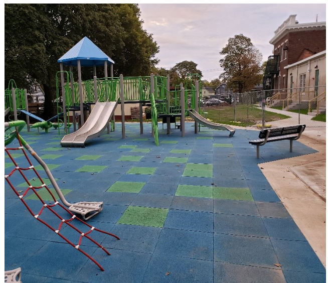
School #25 – Playground replacement project
