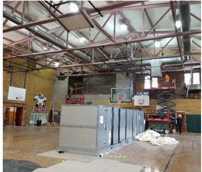
Franklin – Gymnasium air handler unit replacement
